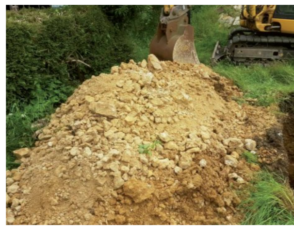
MATERIAL FROM TRAIL PIT PERMEABLE WEATHERED INFERIOR OOLITE
